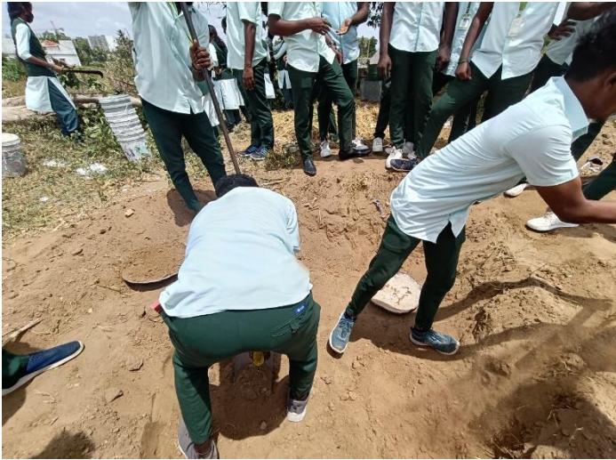
Digging of Compost Pit
